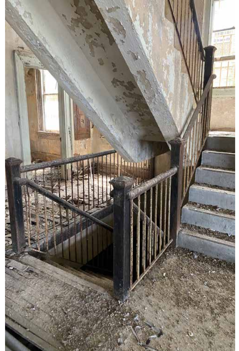
EXISTING SECOND FLOOR STAIR
